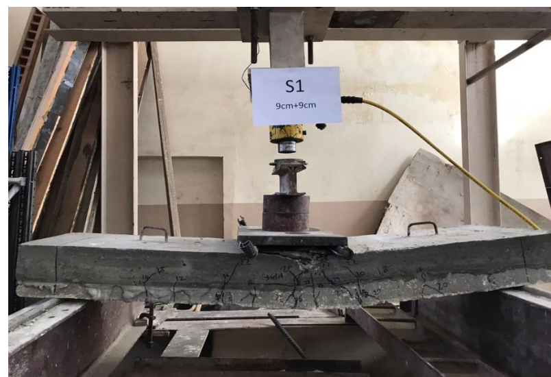
Fig. (5) – “S1” Slab 1 cracks shape
